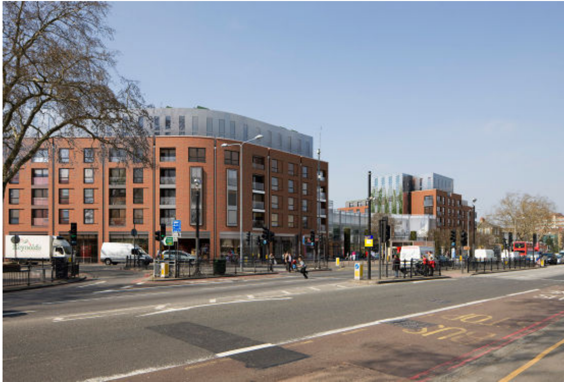
View north-west from High Road
